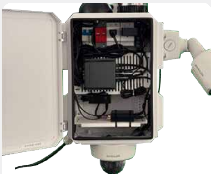
Interior view of the box
